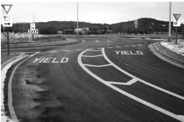
Figure 2-16b: Occasional entry with double white lines separating entry lanes. STH 35 and Hanley Road near Hudson.
